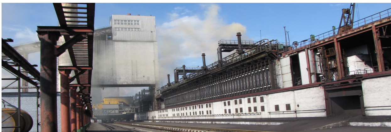
The Alchevsk Coke Plant was the site of a TGF waste heat recovery project. Photo credit: Kari Hämekoski
